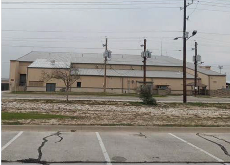
Southwest elevation, viewing northeast.
