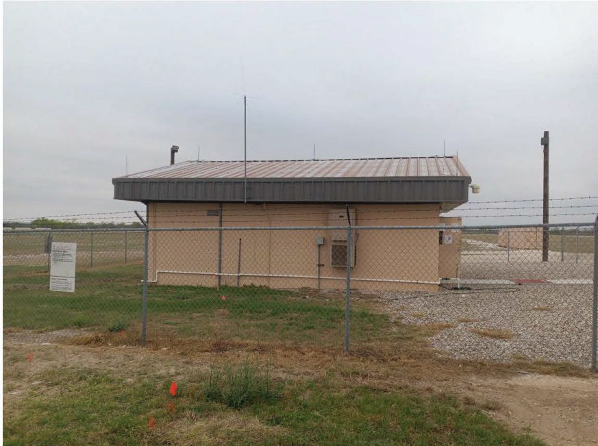
North elevation, view facing south.
