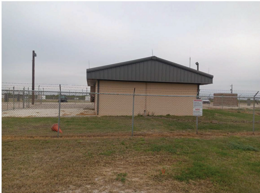
East elevation, view facing west.
