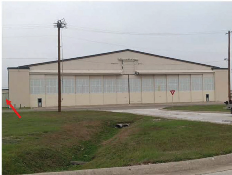
South elevation, viewing north. Note: addition to far left indicated by red arrow.
