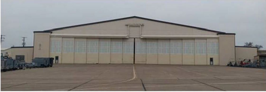
Facade (north elevation). viewing south.
