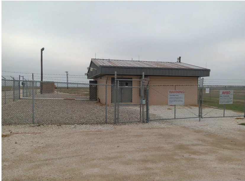
South elevation, view facing north-northeast.
