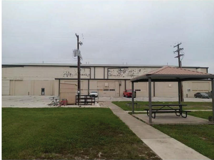
East elevation, viewing west.
