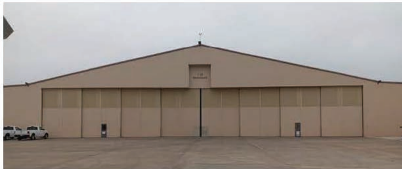
Façade (northwest elevation), viewing southeast.
