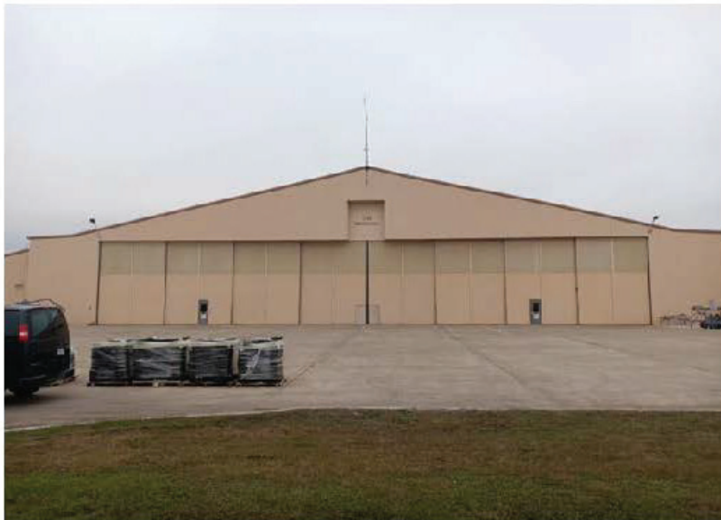
Southeast elevation, viewing northwest.
