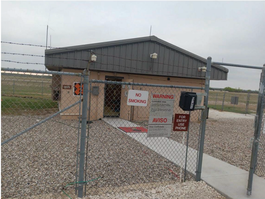
Façade (west elevation), view facing east.
