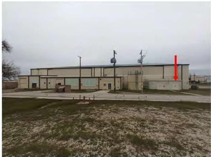
West elevation, viewing east. Note: addition to right indicated by red arrow.
