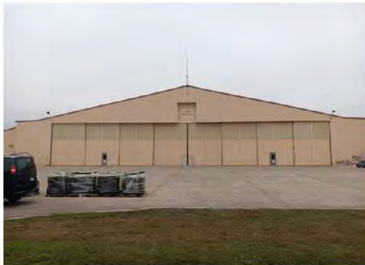
Southeast elevation, viewing northwest.
