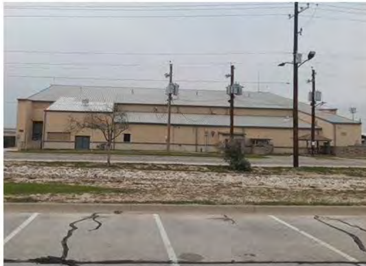
Southwest elevation, viewing northeast.
