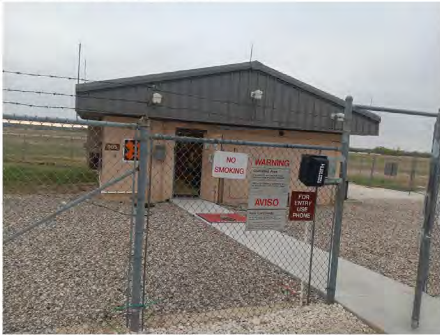
Façade (west elevation), view facing east.
