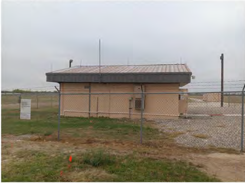
North elevation, view facing south.
