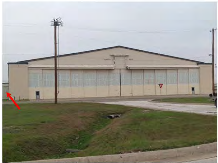
South elevation, viewing north. Note: addition to far left indicated by red arrow.
