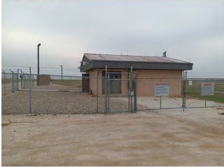
South elevation, view facing north-northeast.
