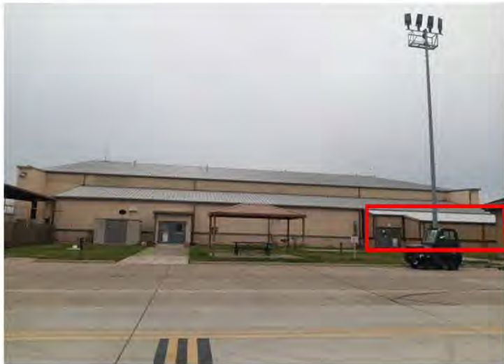
Northeast elevation, viewing southwest. Note: the addition is outlined in red.
