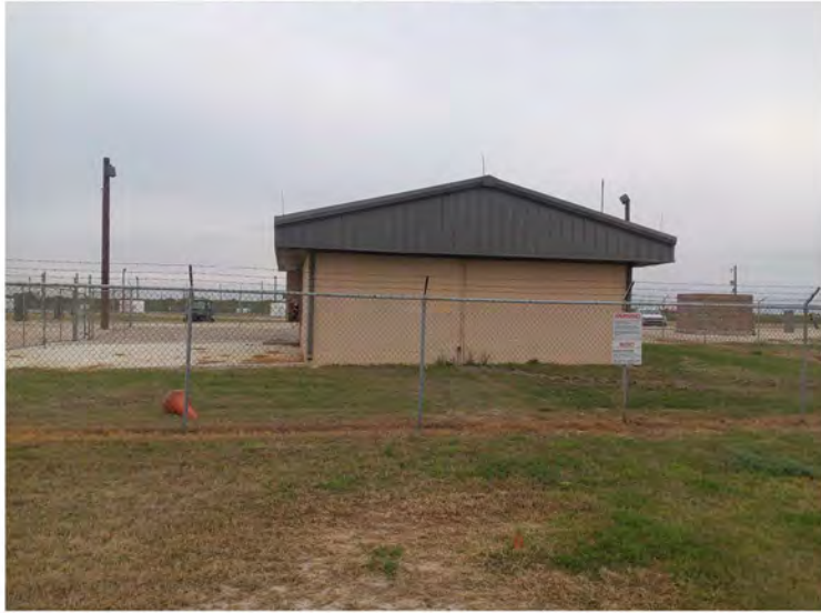
East elevation, view facing west.
