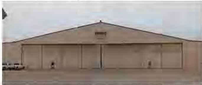
Façade (northwest elevation), viewing southeast.
