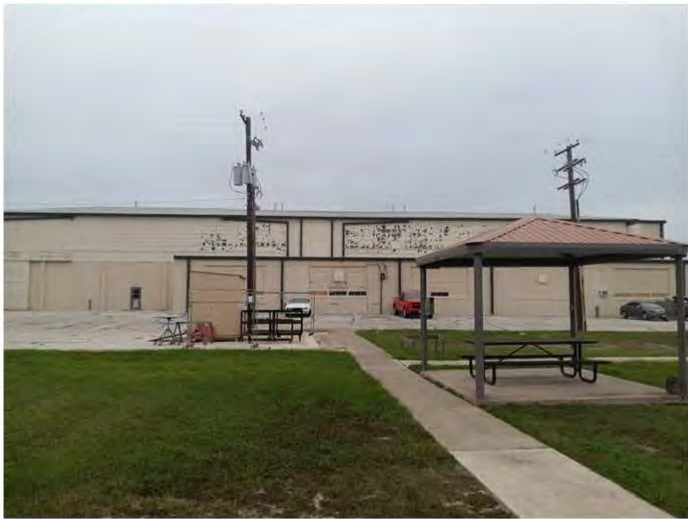
East elevation, viewing west.
