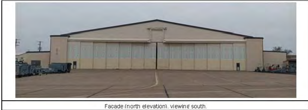
Facade (north elevation), viewing south.
